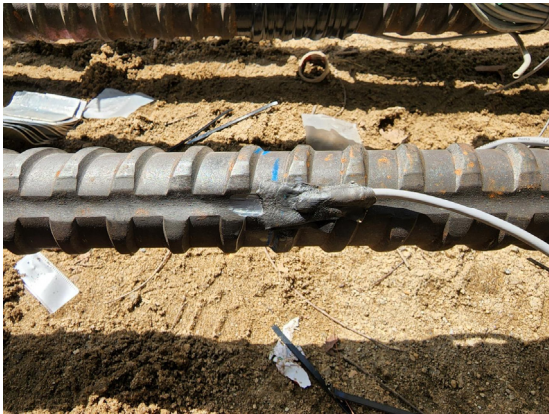
(c) 2nd waterproof coating (Butyl rubber tape)
