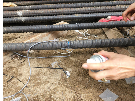
(b) 1st waterproof coating (acrylic coating spray)
