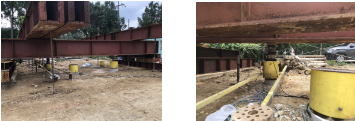
Fig. 12. Field load tests
